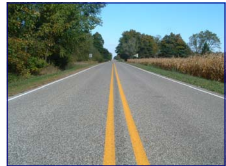
An application of Chip Seal on this Clinton County road will extend the life of the pavement for several years.
